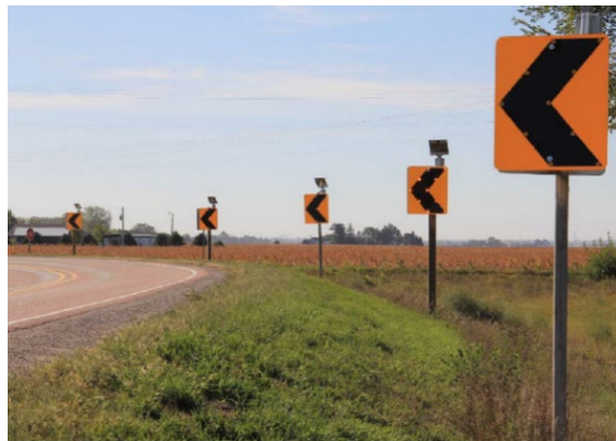
Figure 4. Solar-powered Sequential Dynamic Curve Warning Systems on two-lane roadway. Image from the Pennsylvania Department of Transportation, https://www.penndot.pa.gov/about-us/StateTransportationInnovationCouncil/Innovations/Pages/Lighting-Curves.aspx
