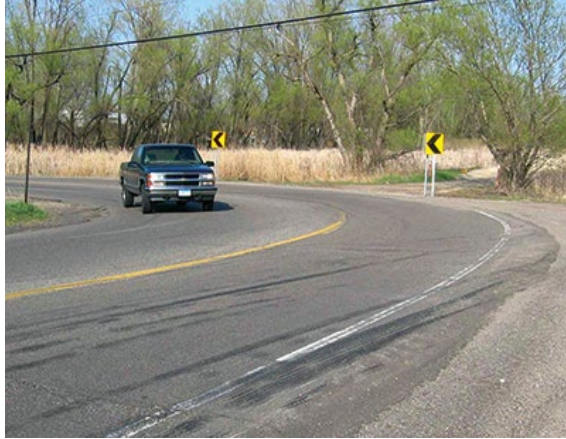
Figure 9. Wide shoulder on horizontal curve.
