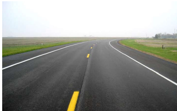
Figure 8. Wide lane on horizontal curve.
