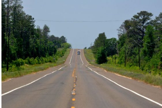
Figure 2. Clear Zone on two-lane roadway.
