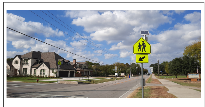
Figure 1. Example of LED-Em treatment at a school crossing. ©2022 Texas A&M Transportation Institute.
