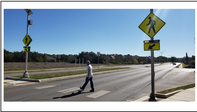
Figure 3. Example of a rectangular rapid flashing beacon (RRFB) treatment. ©2022 Texas A&M Transportation Institute.
